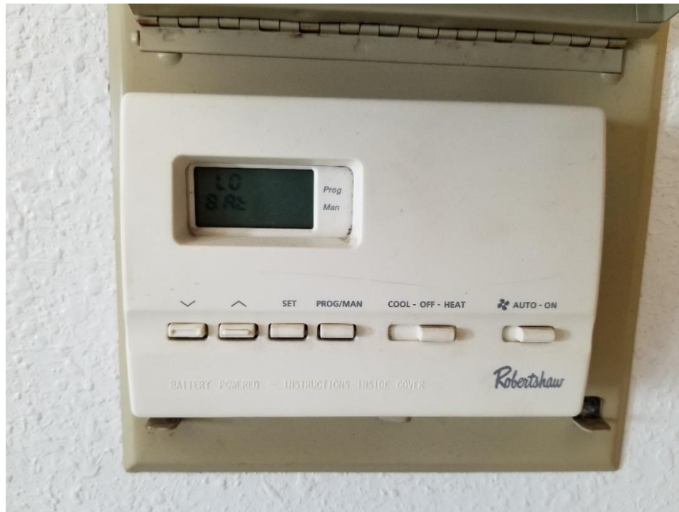
Thermostat in Library not working properly due to low battery. It is recommended to change the battery on this unit or replace it.
