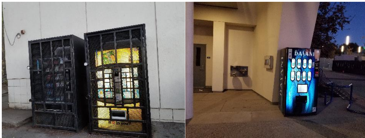
Vending machines throughout Santa Monica HS without occupancy vending misers.
