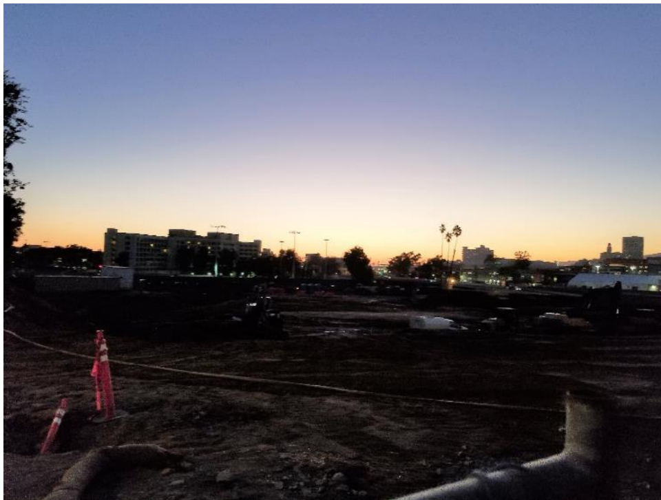
Construction site of new Technology building and parking lot.
