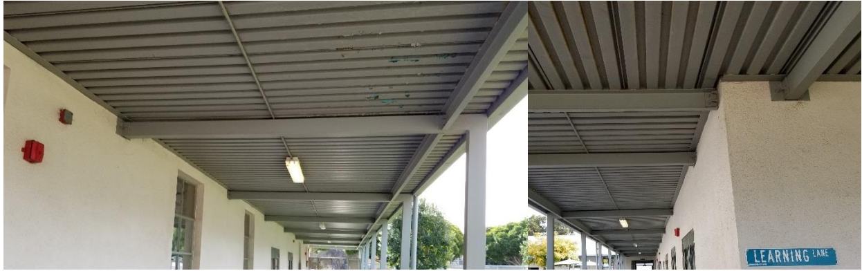
Exterior canopy lights on during the day due to a possible issue with the timer controls
