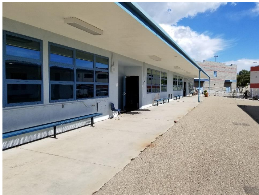
Classrooms with large windows but without curtains. During the fall and summer, these classrooms tend to heat up due to the large window area. It is recommended to add curtains to save on cooling during the warmer months.
