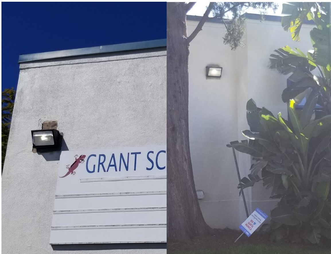
Exterior lights on during the day due to a possible issue with the timer or photocell.
