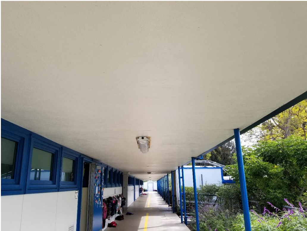
Recently retrofitted exterior lights with photocell sensors.
