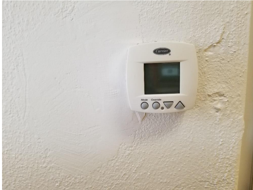
Thermostat in Faculty workroom not working properly. It is recommended to change the battery on this unit or replace it.
