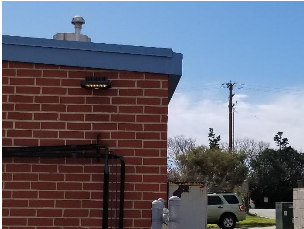
Exterior lights on during the day outside of cafeteria and classroom buildings, possibly due to broken photocell or timer controls.
