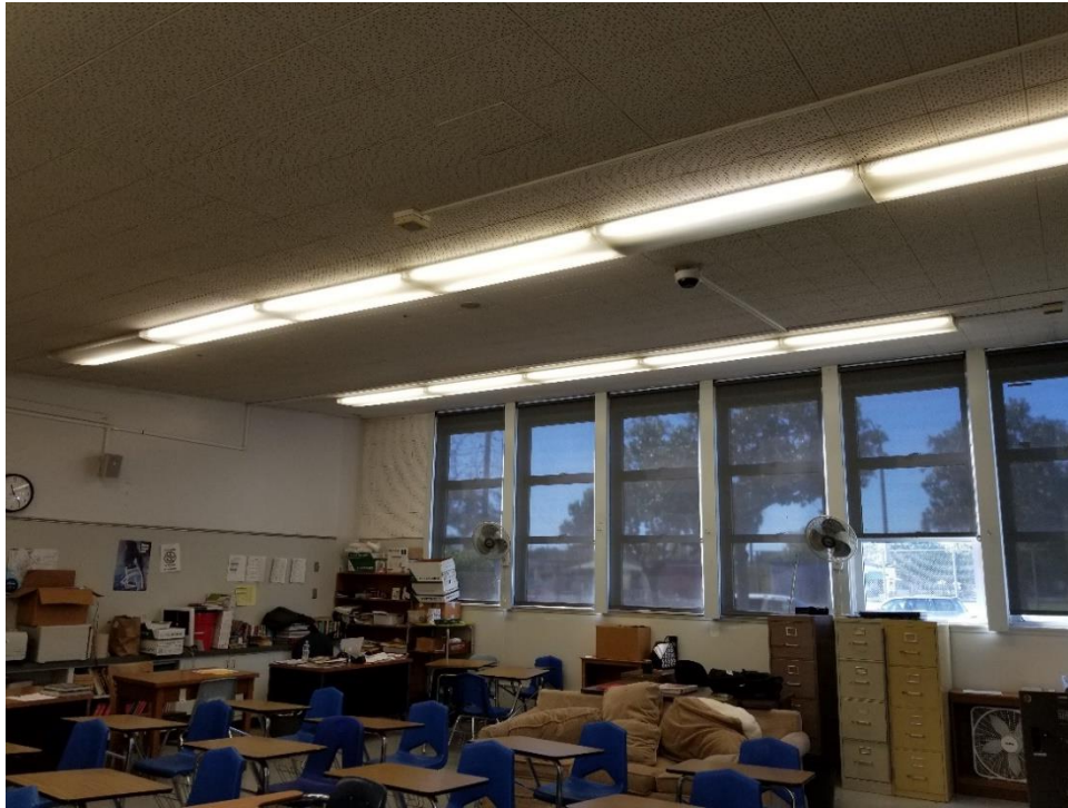
Classroom with shades on windows. This is recommended, especially in the fall and summer, in rooms with a large window to wall ratio to reduce radiant heat.
