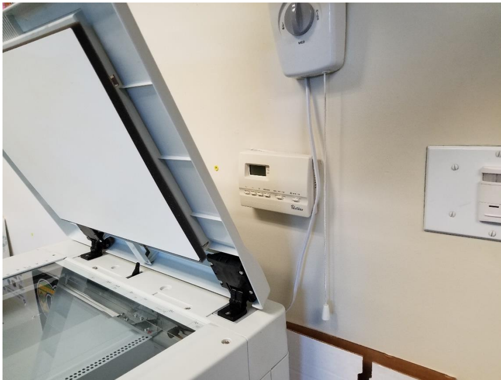
Thermostat in office next to copier not working properly due to low battery. It is recommended to change the battery on this unit or replace it.
