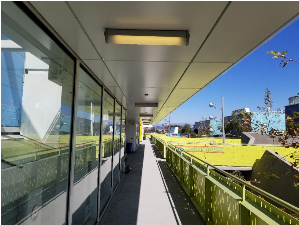
Exterior lights on during the day due to a possible issue with the timer or photocell.
