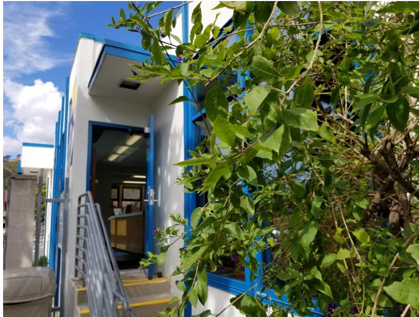
Office backdoor left open while the heater was set to 85°F. It is suggested to close doors while the heater is running or turn down the set-points to more reasonable levels.
