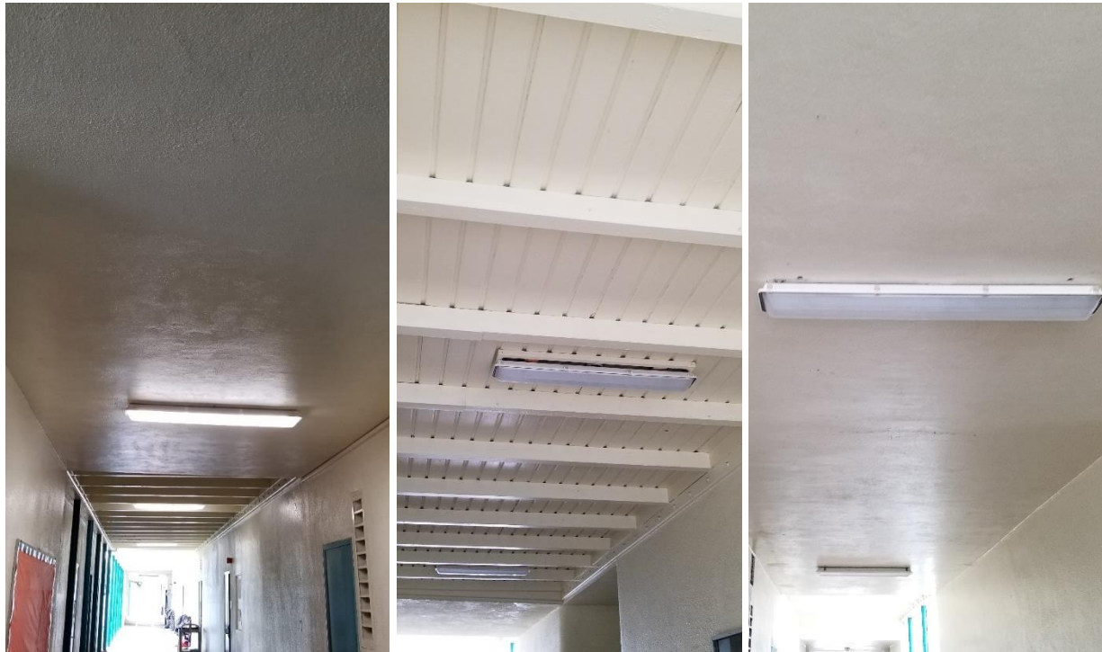
Exterior canopy lights on during the day. It was mentioned that in the longer hallways, lights are left on for safety purposes. However, there were other lights that were not on and daylight appeared to adequate. It is therefore recommended to turn off these lights during the day.
