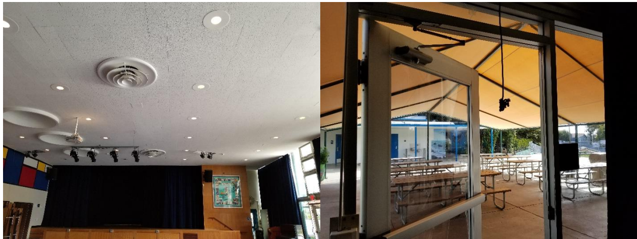
Lights left on in Multipurpose Room/Cafeteria with large windows and curtains. This room could save significant energy in that during the winter, curtains can be opened so that electrical light is not necessary and during the summer and fall, curtains can be closed to block out radiant heat and save on cooling.
