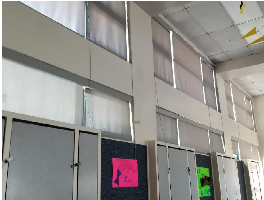
Cafeteria with large windows and curtains. This room could save significant energy in that during the winter, curtains can be opened so that electrical light is not necessary and during the summer and fall, curtains can be closed to block out radiant heat and save on cooling.
