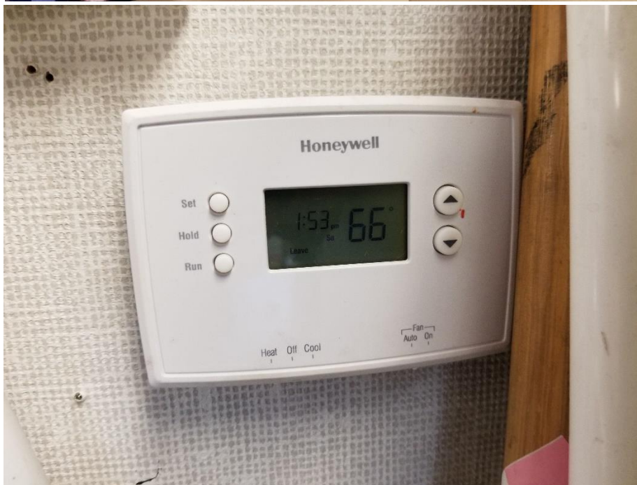
Thermostats programmed on the wrong date and time. If a thermostat is running a program, it is recommended to check at regular intervals that time and dates are correct.
